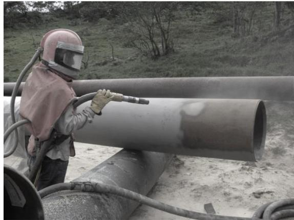
*Fig (2) shows a person carrying out sandblasting*
